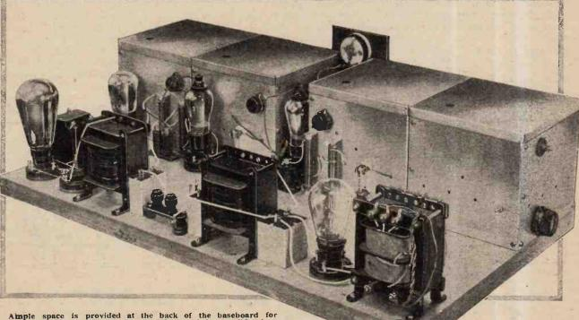
Ample space is provided at the back of the baseboard for assembling the mains equipment while permitting modifications to be made to the L.F. amplifter and output stage as may be indicated by subsequent progress and more ambitious requirements.
